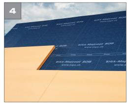
Lay diffusion-open thermal insulation above Majcoat (SOB) ≥ 52 mm
