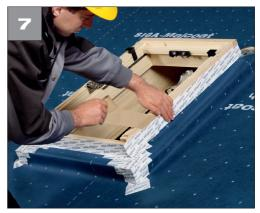
Seal the roof underlay membrane all round the skylight frame so that it is windtight
