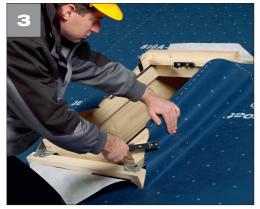
Secure the roof underlay membrane to installation and skylight frame on all sides
